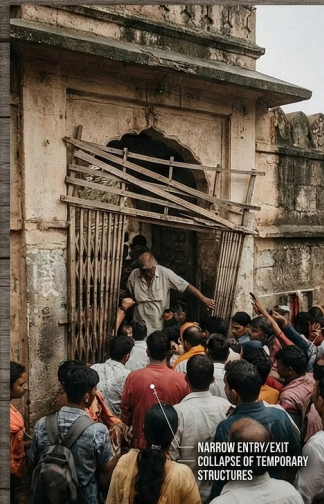
PANEL 2: STRUCTURAL DEFICIENCIES | ILLIYAS ET AL. (2013)
